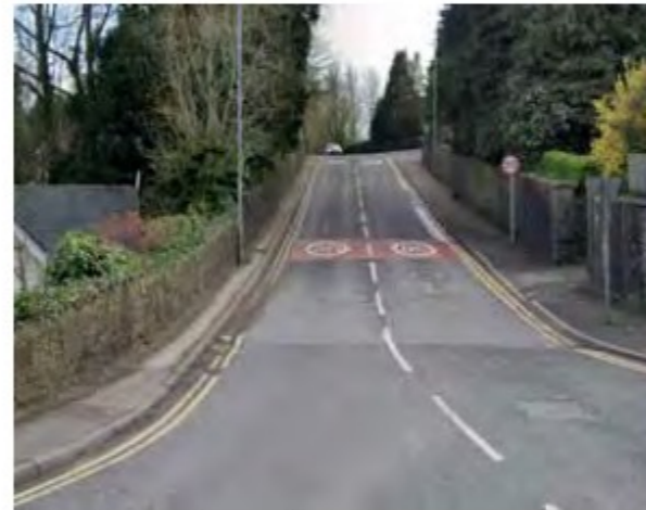
Narrow footways on busy road
