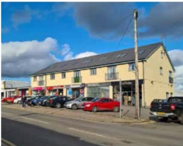
Bulwark shops neighbourhood centre
